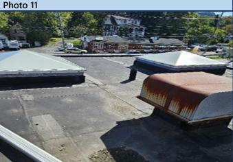
Area B-1960 Roof (@ Front Entrance) ACM Curb Flashing At Skylights
