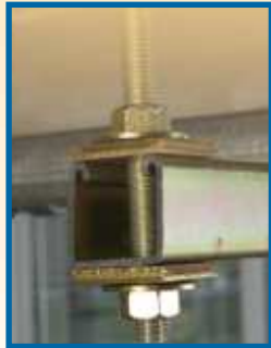
Standard method using nuts and washers.
