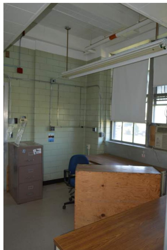
OFFICE (IN-24 DG-101)
