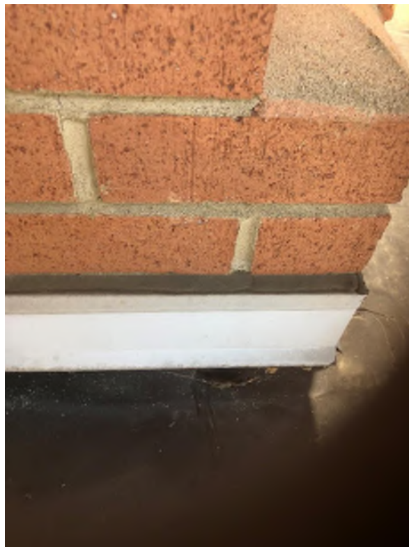
Caulk Around Metal Flashing
