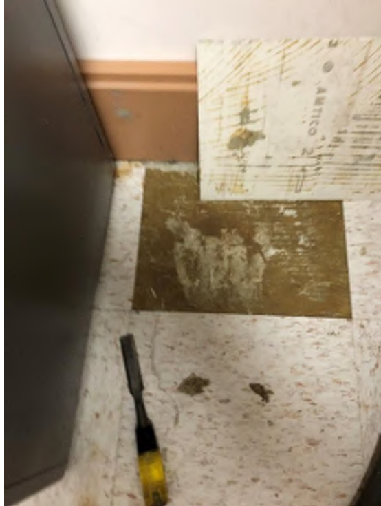
Mastic Under 12x12 with Brown Streaks
