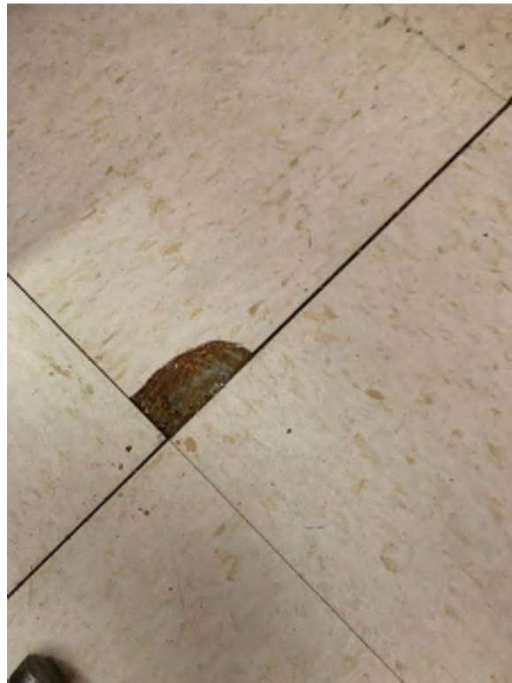
Mastic Under Yellow Streaks Tile
