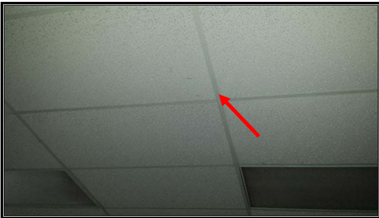
Photo # 04: 2'x4' Gouged Ceiling Tile, White
