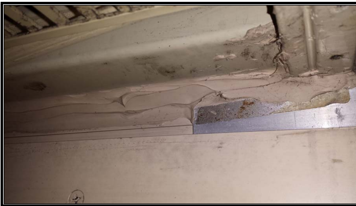
Photograph 8: Interior Window Frame Caulk, Beige (To A/C Units)
