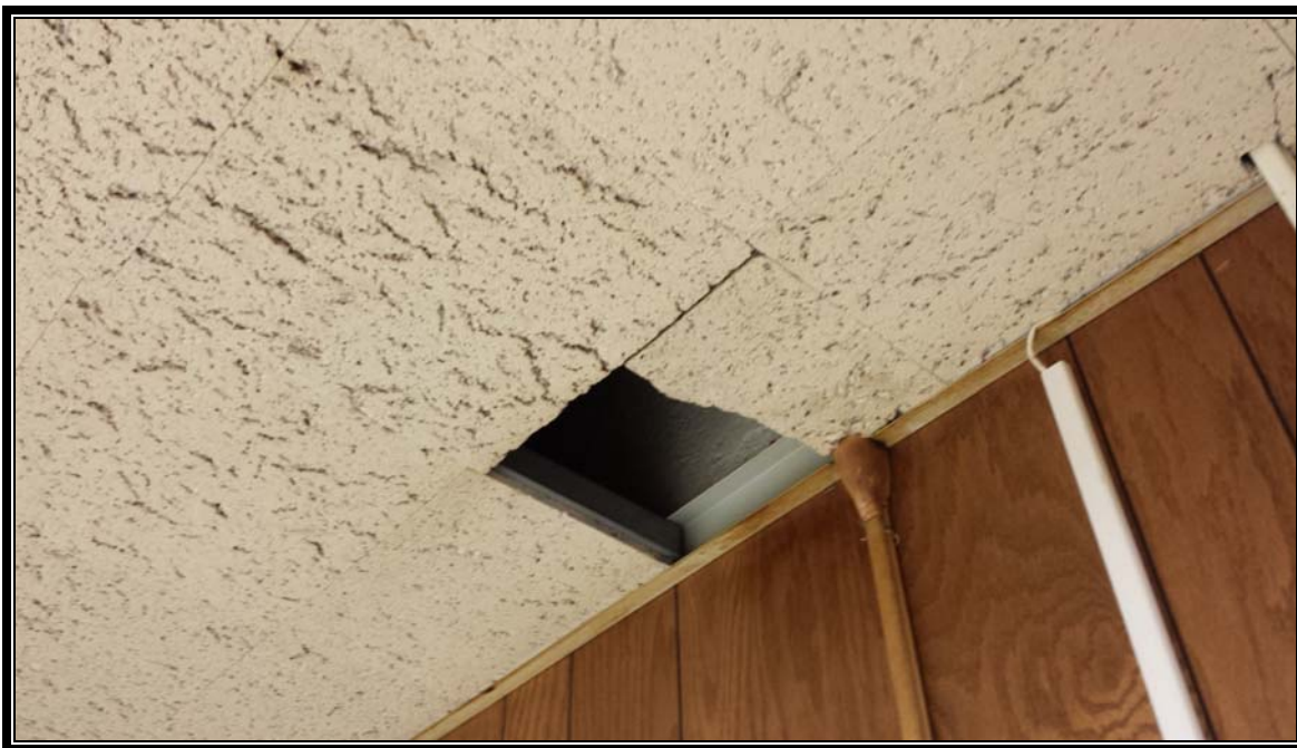
Photograph 9: 1'x1' Ceiling Tile, Spline
