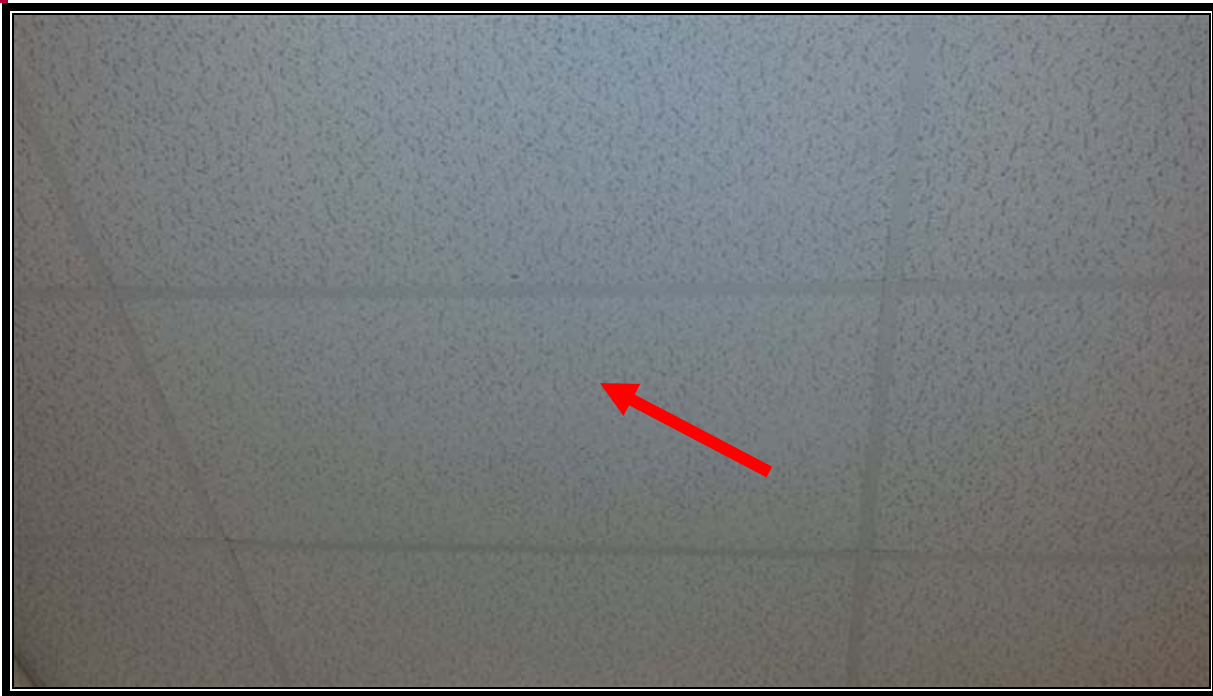
Photo # 05: 2'x4' Fissured/Pinhole Ceiling Tile, White
