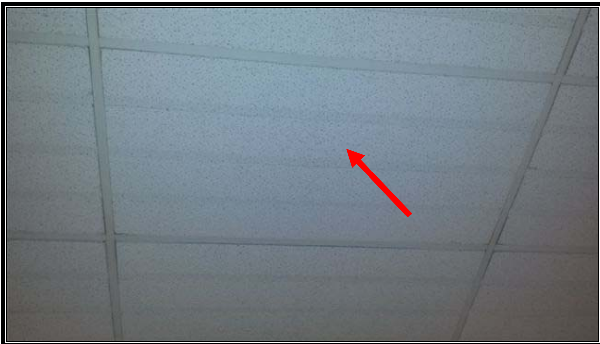
Photo # 06: 2'x4' Stripe Design Ceiling Tile, White
