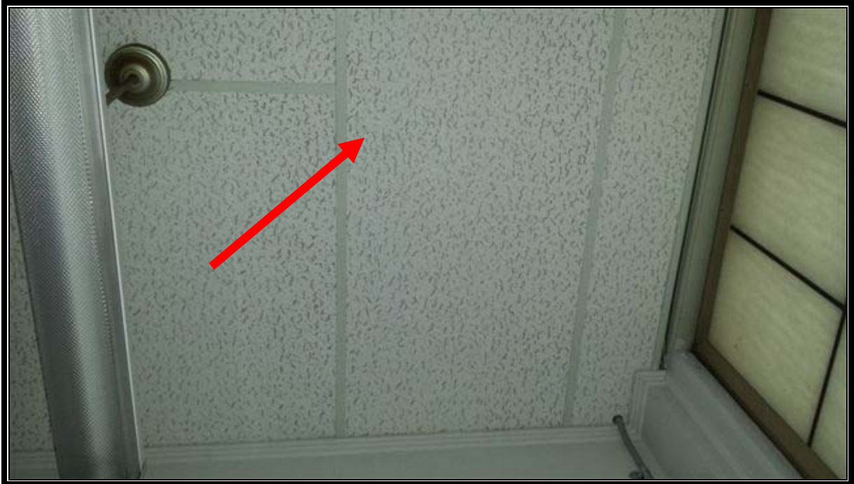
Photo # 01: 2'x4' Large Gouged Ceiling Tile, White
