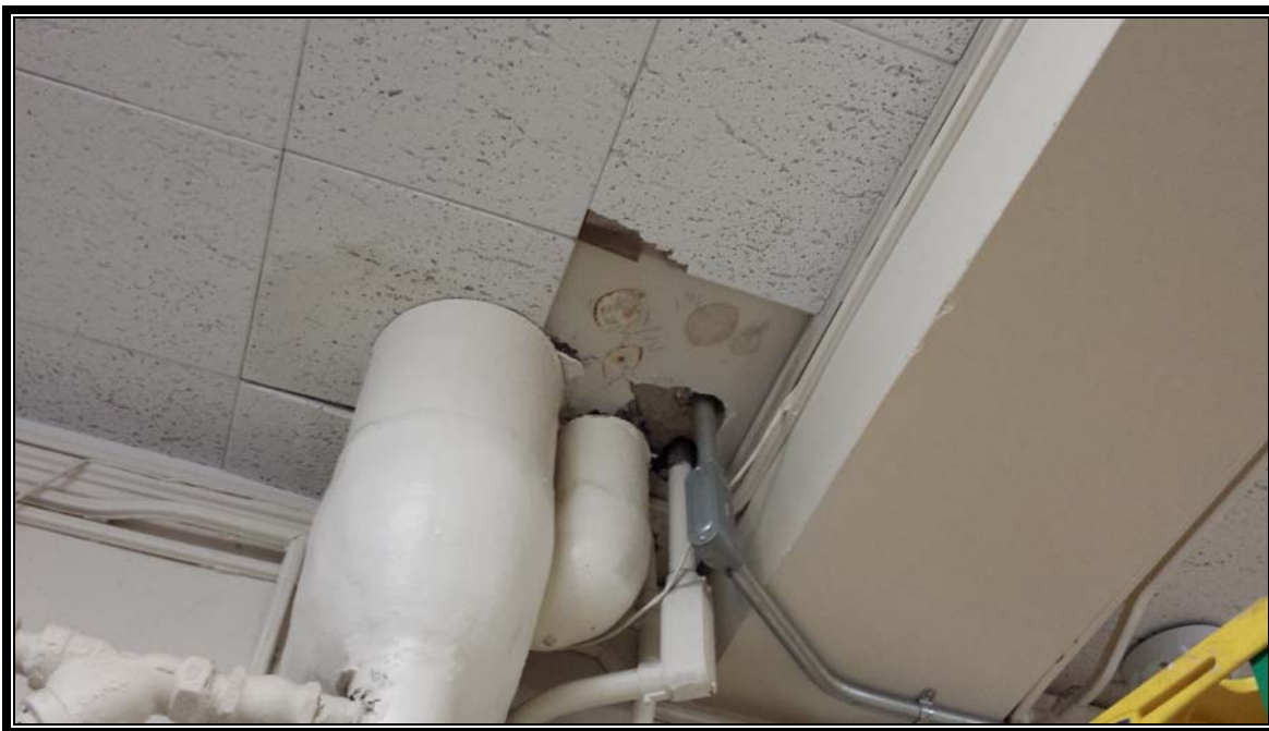
Photograph 3: 1'x1' Ceiling Tile, Textured, 1'x1' Ceiling Tile, Textured, Mastic & Ceiling Plaster, White & Brown Coats
