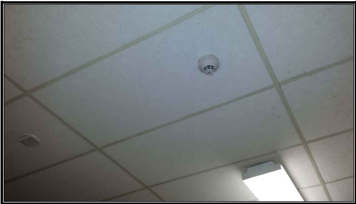
Photograph 5: 2'x4' Ceiling Tile, Patterned/Pinhole
