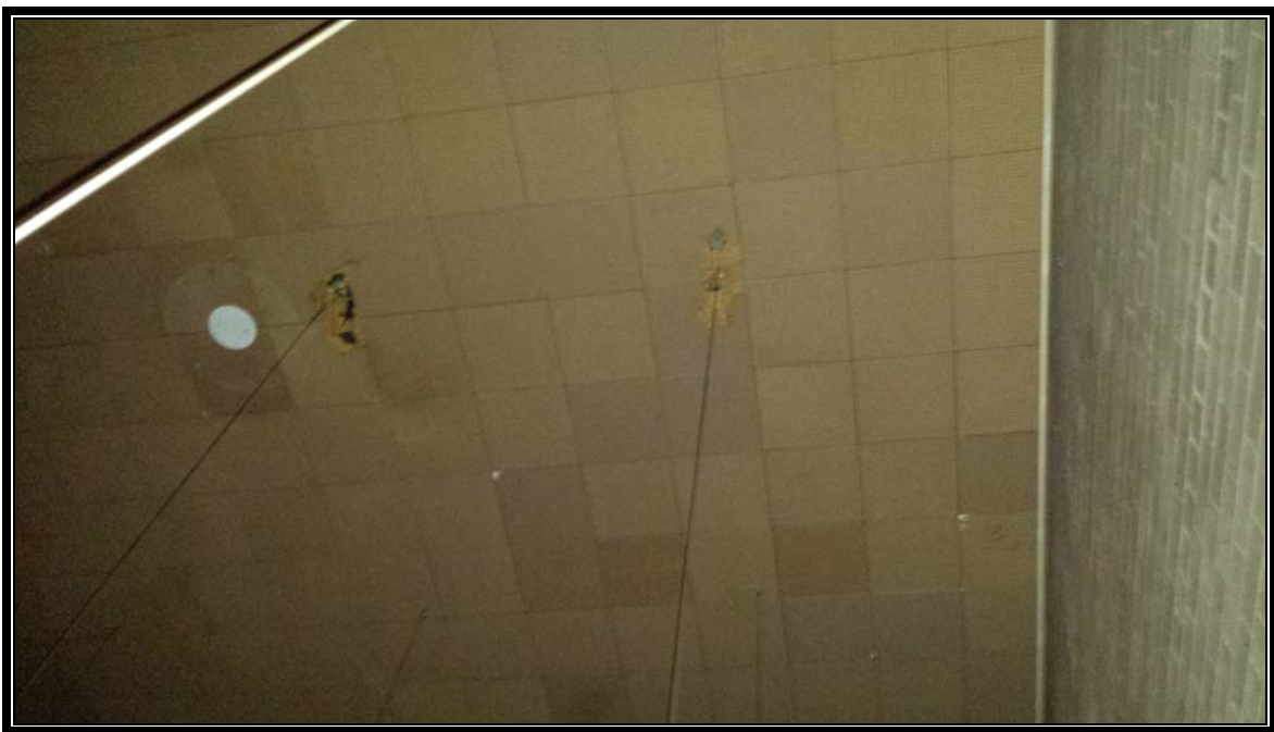
Photograph 6: 1'x1' Ceiling Tile, Pinhole
