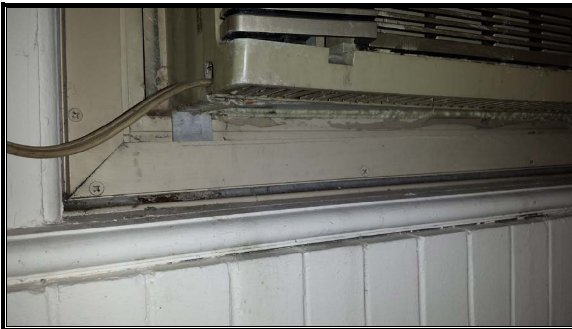
Photograph 7: Interior Window Frame Caulk, Grey
