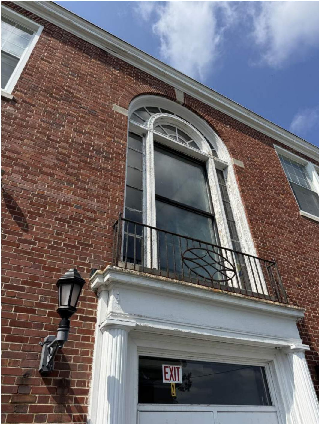
Above: South West Stairwell Window Frame
