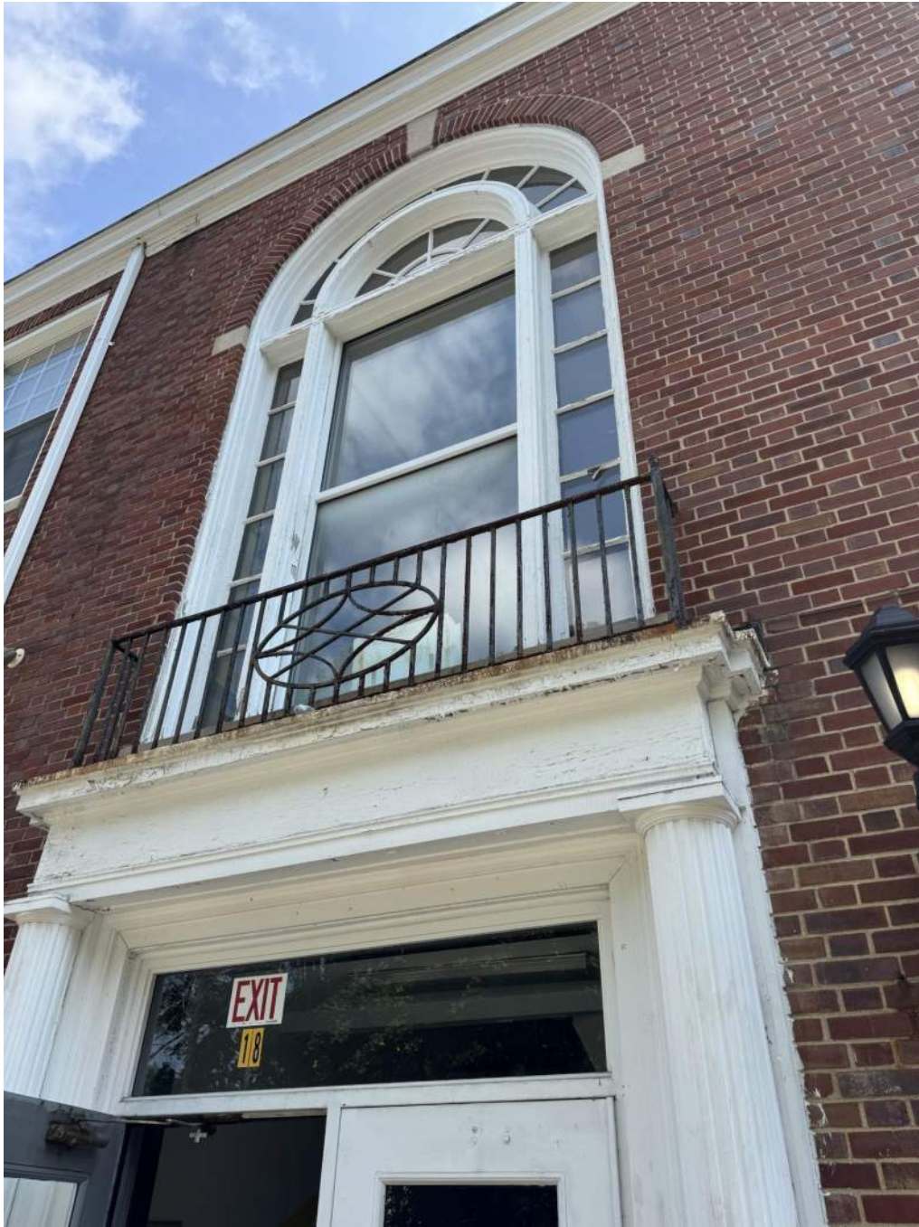
Above: East Stairwell Window Frame
