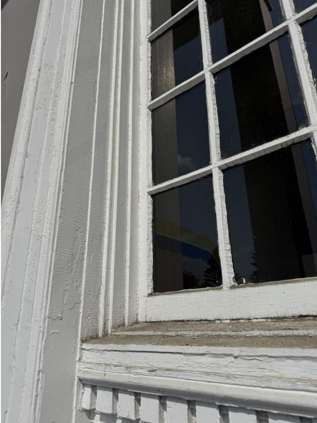
Above: Main Entrance Window Frame
