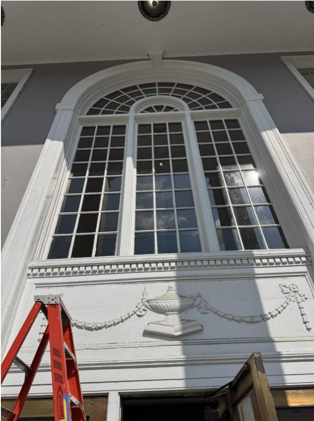
Above: Main Entrance Window Frame
