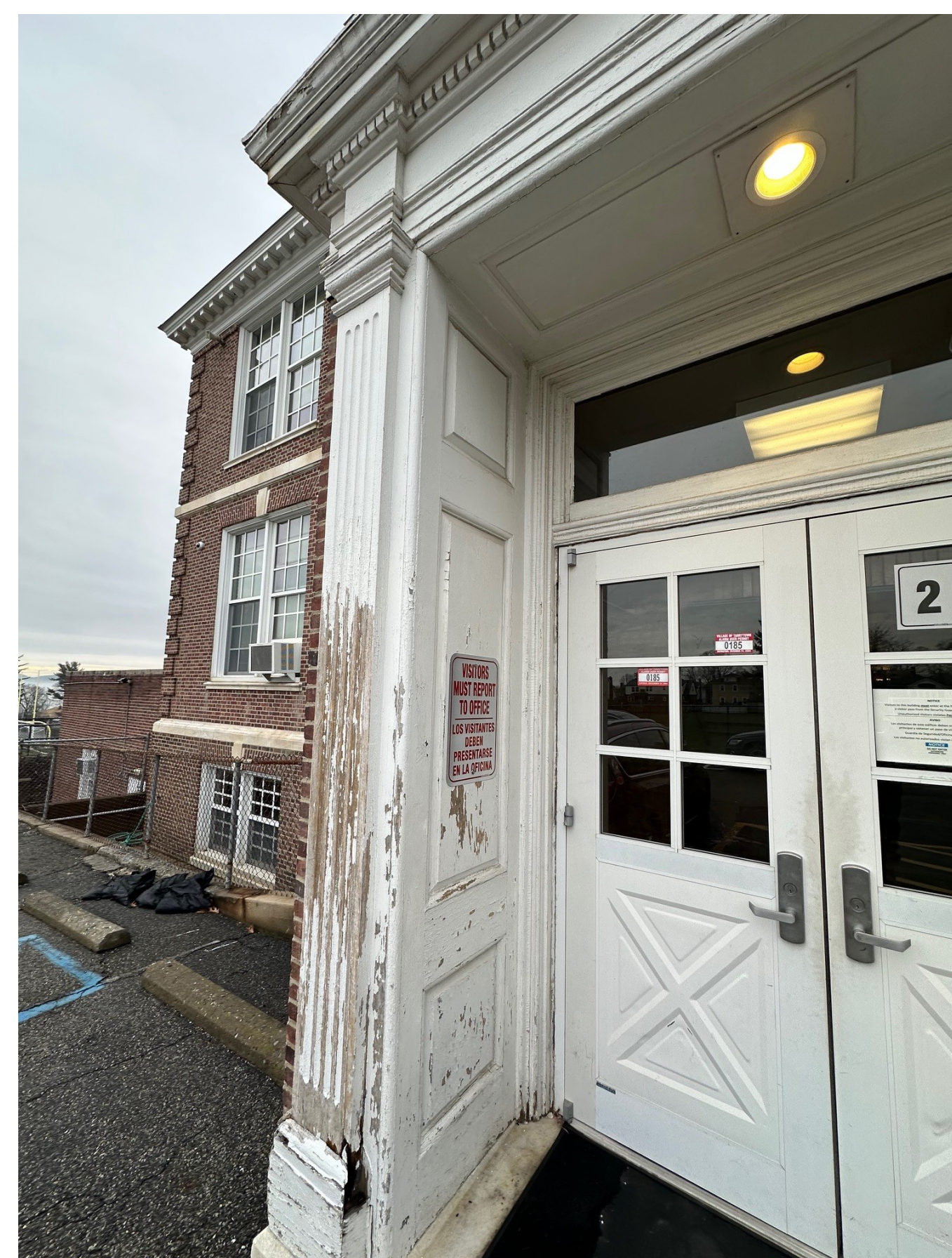
SOUTH ENTRY REFERENCE PHOTO - WEST
