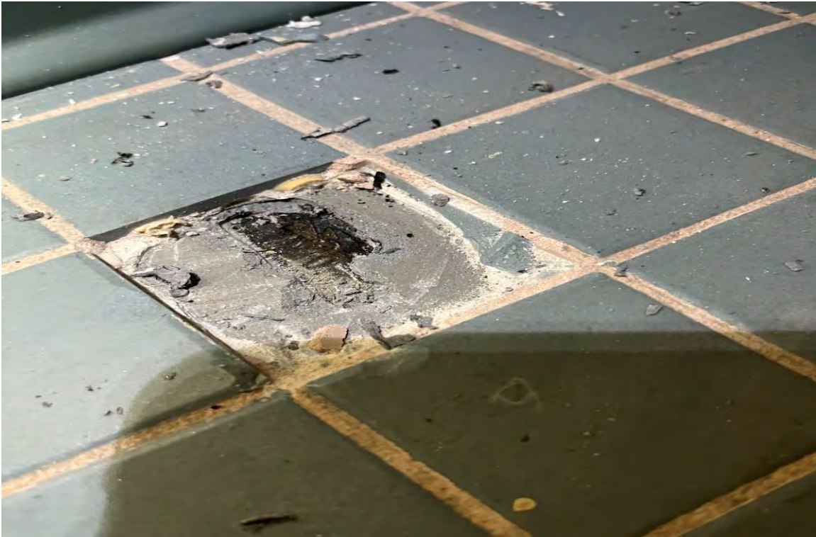
ABOVE: SECOND FLOOR, OFFICE CLOSET – ACM SECOND LAYER FLOOR TILE & MASTIC BELOW: FIRST FLOOR – ACM SECOND LAYER FLOOR TILE (TYPICAL)
