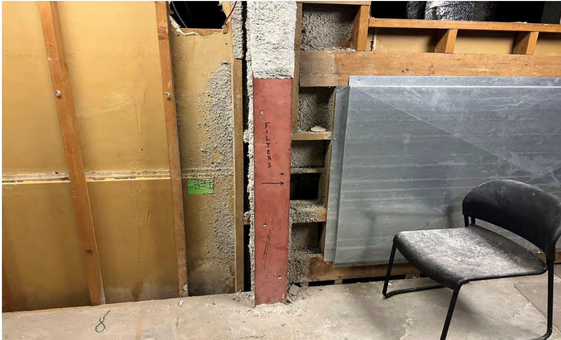
ABOVE: LBP Structural Beam
