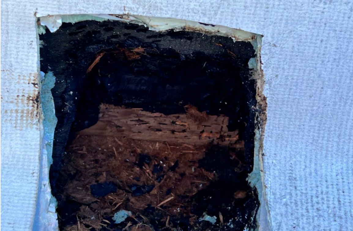
ABOVE: ACM TAR ON PARAPIT & ACM BUILT UP ROOF (PERIMETER) BELOW: ACM TAR & TAR FLASHING ON VENT STACK
