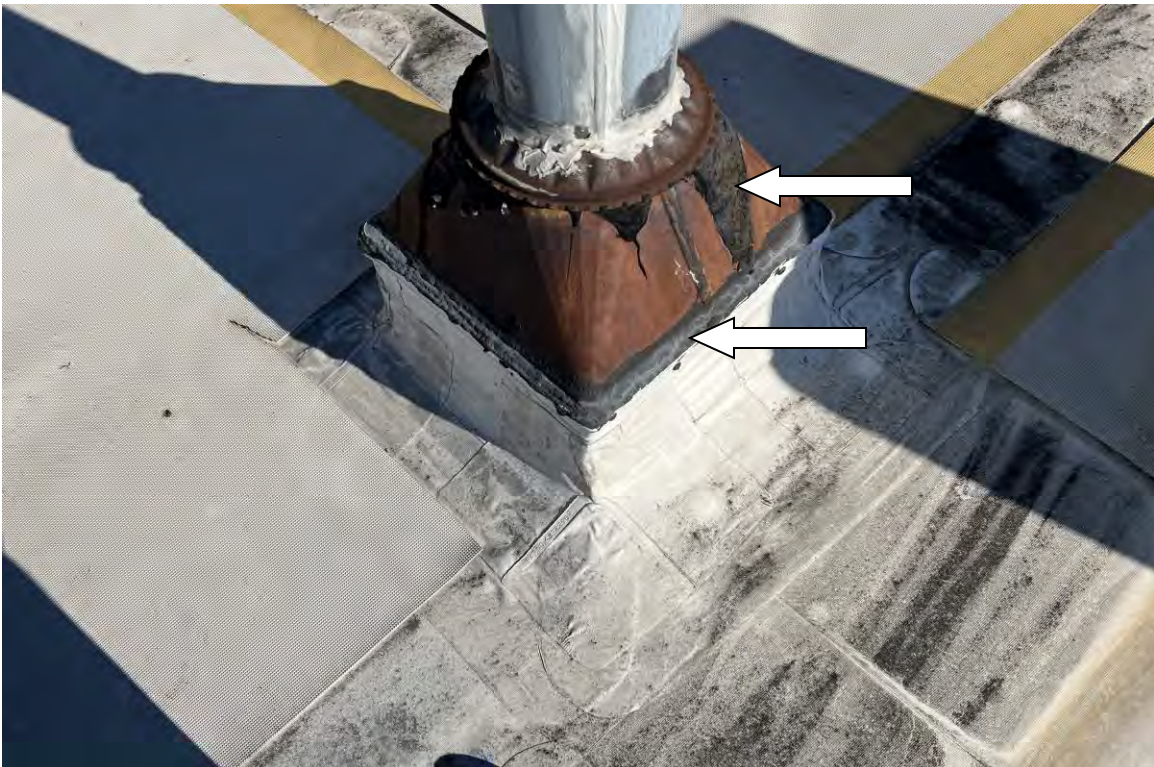
ABOVE: ACM TAR ON PARAPIT & ACM BUILT UP ROOF (PERIMETER) BELOW: ACM TAR & TAR FLASHING ON VENT STACK
