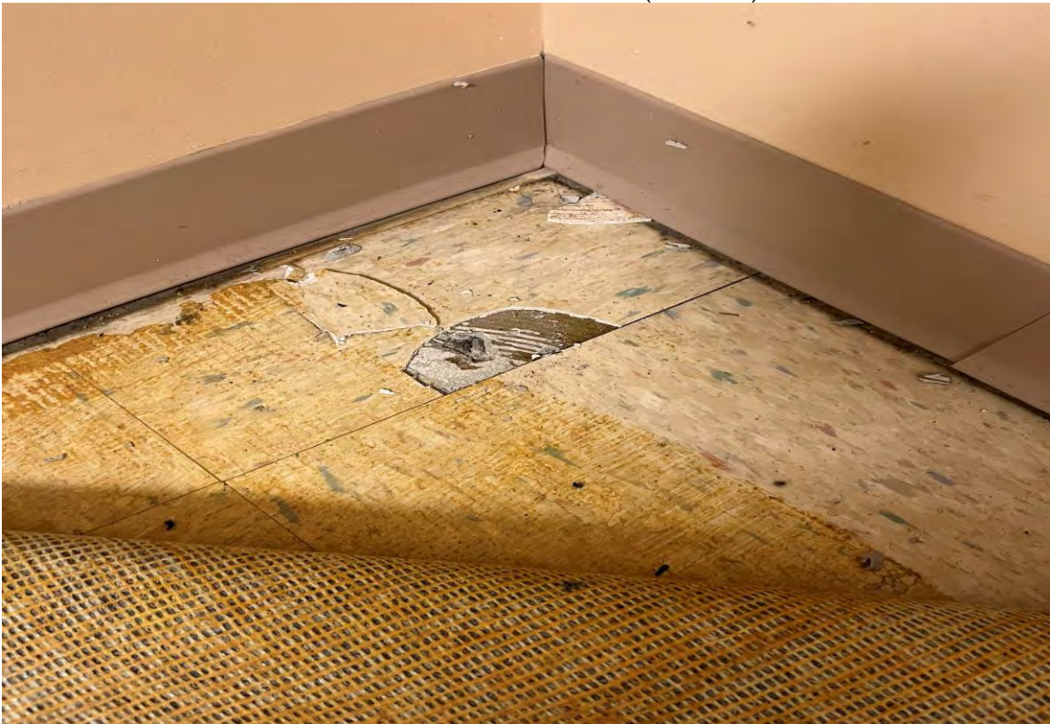
ABOVE: SECOND FLOOR, OFFICE CLOSET – ACM SECOND LAYER FLOOR TILE & MASTIC BELOW: FIRST FLOOR – ACM SECOND LAYER FLOOR TILE (TYPICAL)
