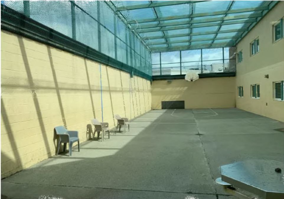
ROOM - RECREATION YARD B
