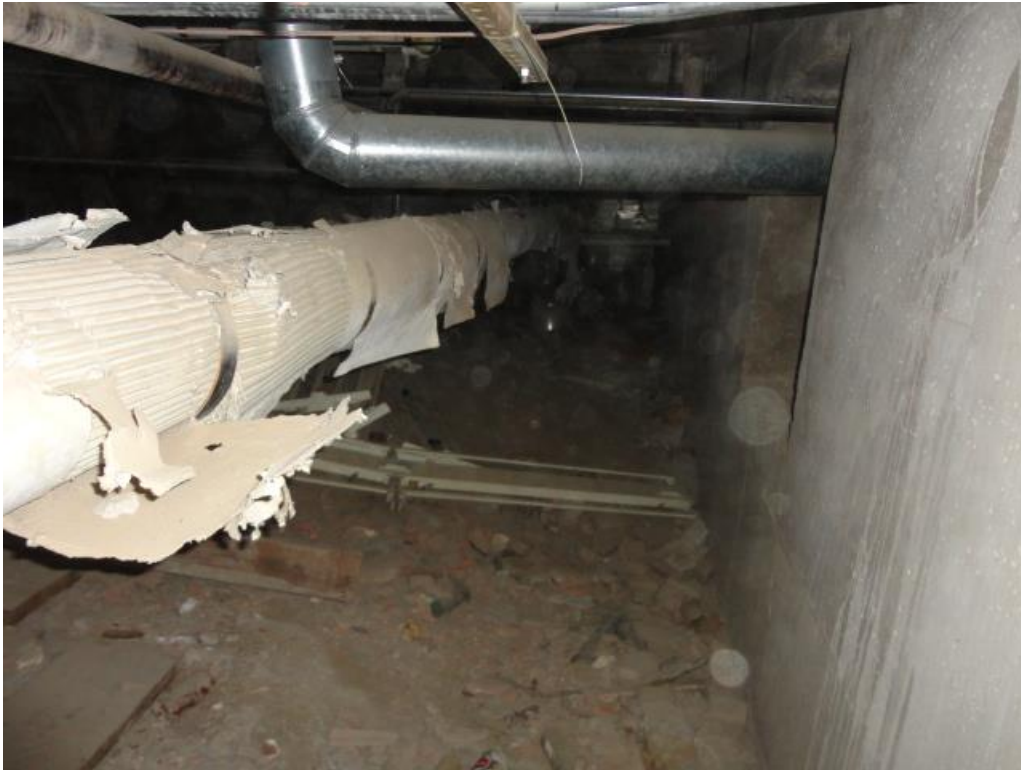
Sample#1 - Air Cell Pipe Insulation - 44.4% Chrysotile
