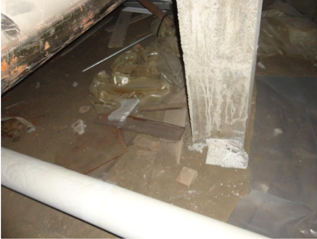
Sample #11 - Debris Location 2 (See Map) - 36.4% Chrysotile & 9.1% Amosite
