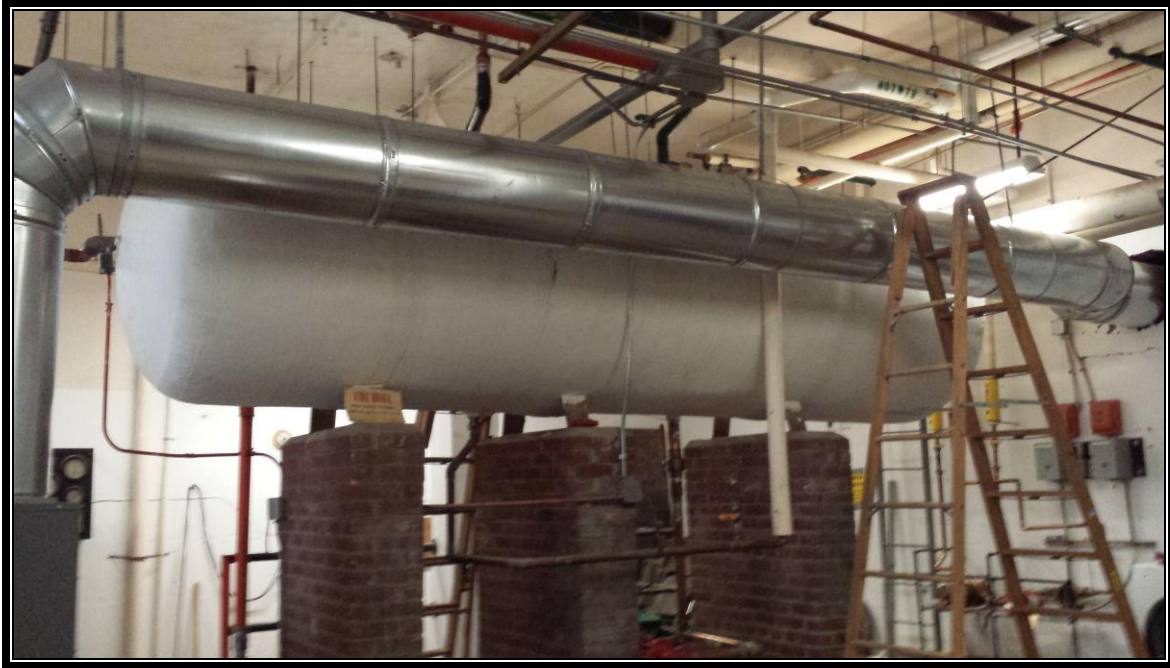
Photograph 3: Water Tank Brick Mortar
