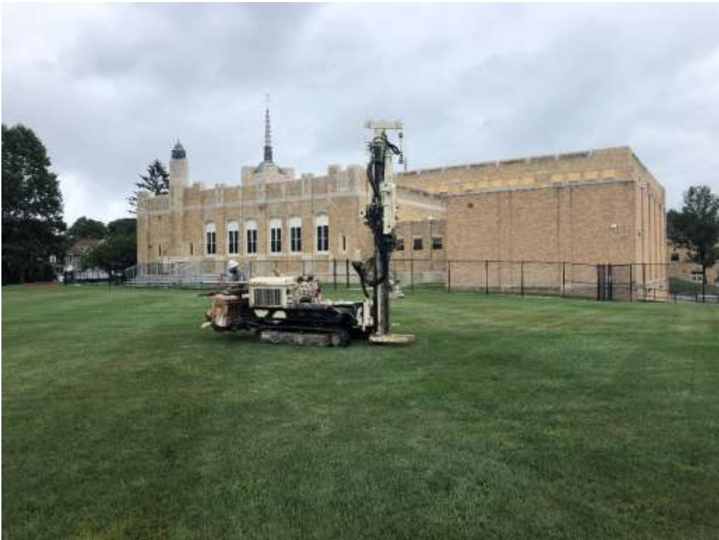
FACING NORTHEAST, TOWARDS B-6 BORING LOCATION.
